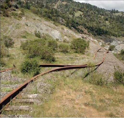
North Coast Railroad Authority Existing Rail
